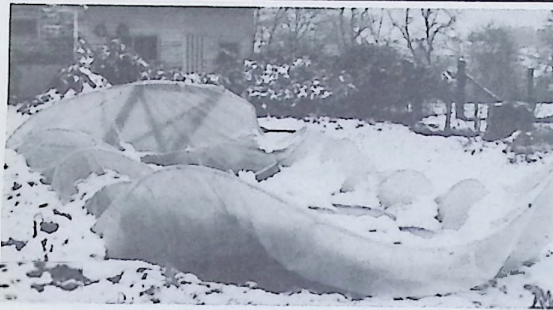
Hoop houses, like this one made with PVC piping for ribs and covered with polyfilm, are meant to be temporary structures, and this one was. It lasted all of five days before snowload caused it to collapse.
